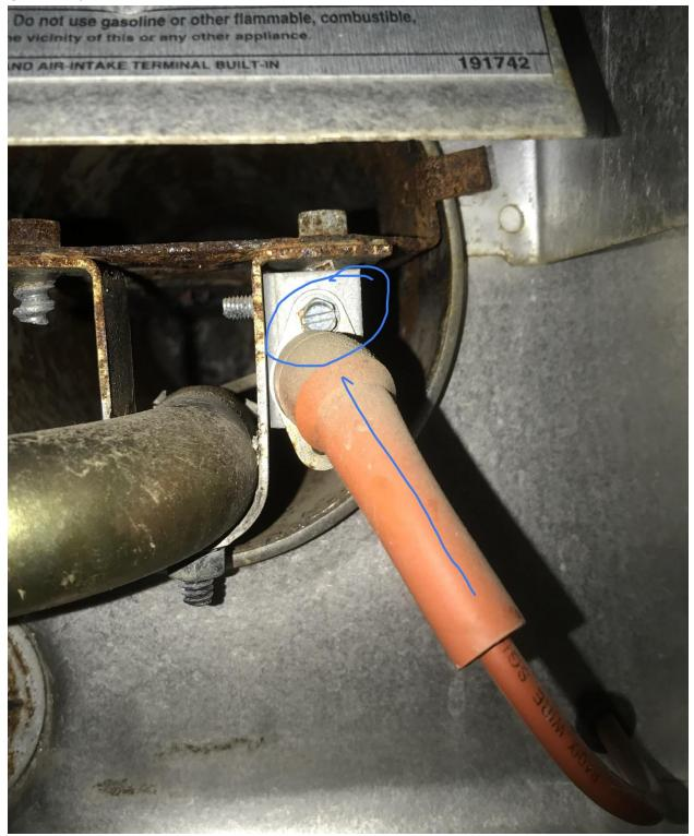
To remove the igniter simply remove 1 bolt circled in Blue.. slide the assembly out and inspect electrode for corroded or sooted up condition.. clean with steel wool being careful not to disturb the position of flame sensor electrode
