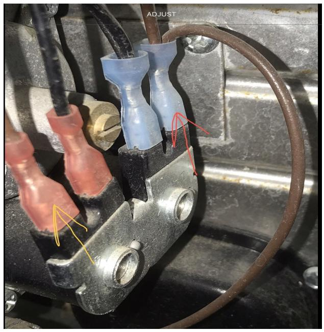
Remove wire marked with yellow arrow.. place multimeter in DC scale. Touch Red lead from meter to wire connector removed and Black meter lead to a ground on the water heater...
