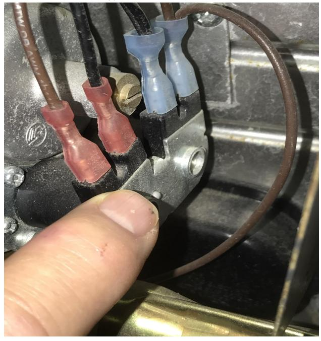
If you don't "feel a thunk" we can isolate whether you have an issue of NO 12 volts DC to one of the solenoids OR both and we can also verify both solenoids are either good or bad..
