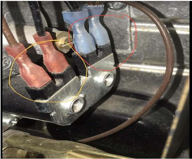
Remove BOTH connections from solenoid circled in yellow..remember which connector went where..
