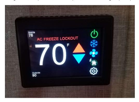
Bedroom, Set point 68, room temp 74, unit not running, required power cycle to reset
